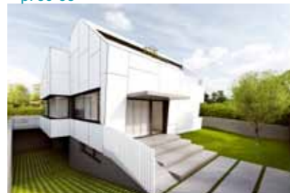
Single-family house #1412 BARCELONA, SPAIN > p. 60-63
