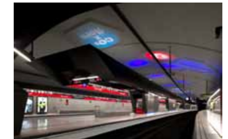
Sant Andreu Metro Station Reform BARCELONA, SPAIN > p. 112-115
