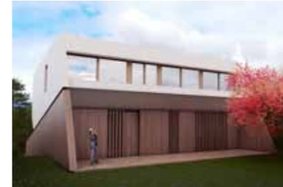
Single-family house #1508 BARCELONA, SPAIN > p. 92-97
