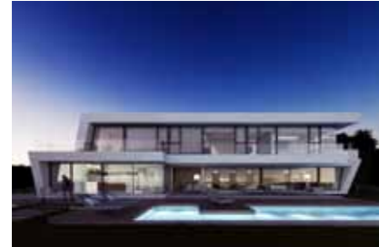
Single-family house #1510 BARCELONA, SPAIN > p. 28-39
